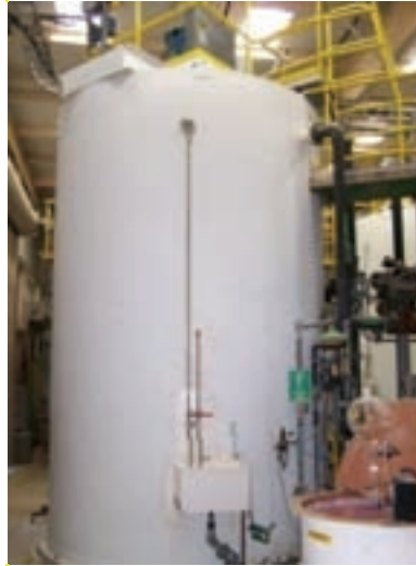
This "solids contact treatment" system processes 17.5 gallons per minute, increasing overall water recovery for reverse osmosis.
