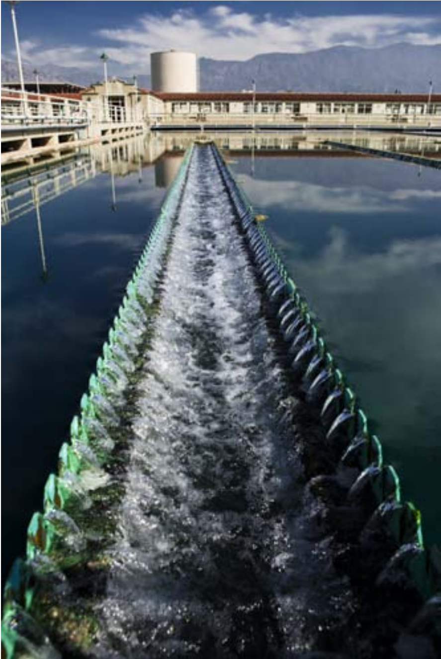
Water flows from Sedimentation Basin No. 3 at the F.E. Weymouth Water Treatment Plant, as solids are skimmed from the surface prior to being filtered. Filter Building No. 1 is in the background.
