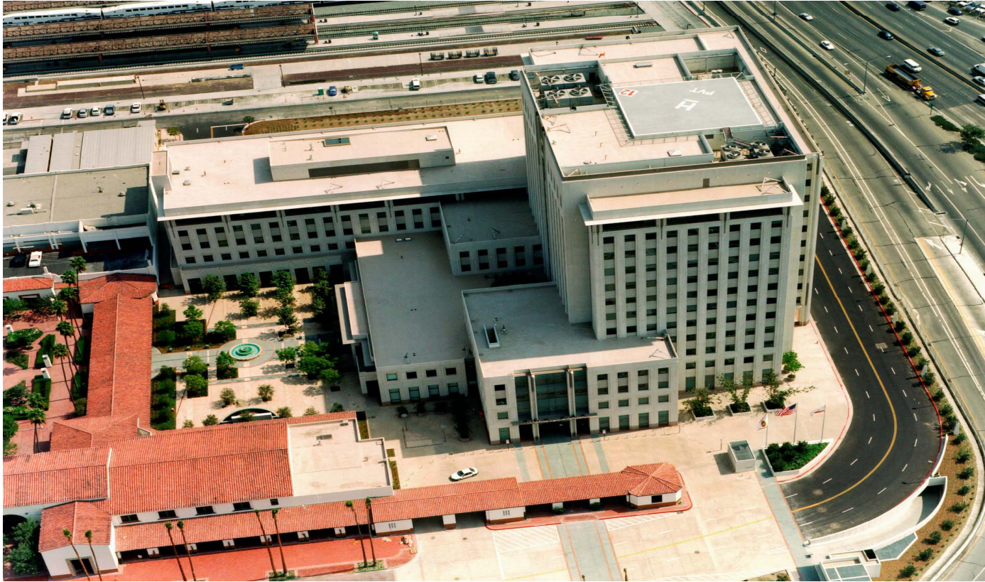
In operation since Fall 1998, Metropolitan's Union Station headquarters houses more than 900 employees. Its proximity to a major transportation hub has triggered a surge in ridesharing among MWD staff.
